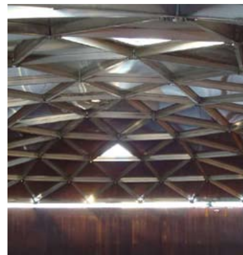
Underside view of skylights
