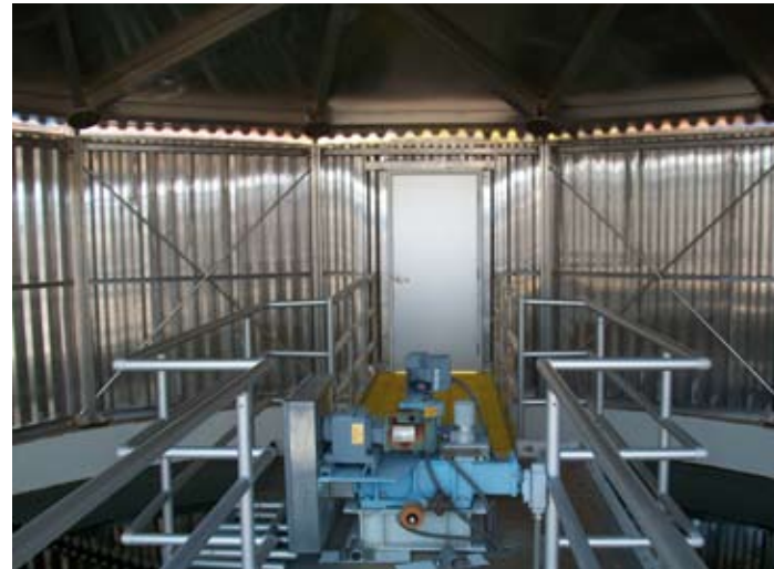
Inside view of sidewalls
